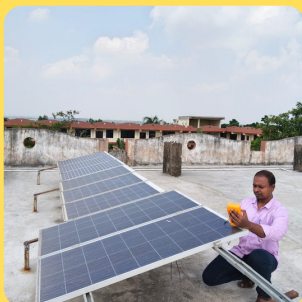
1 kw Solar panel erected and commissioned in our college campus
